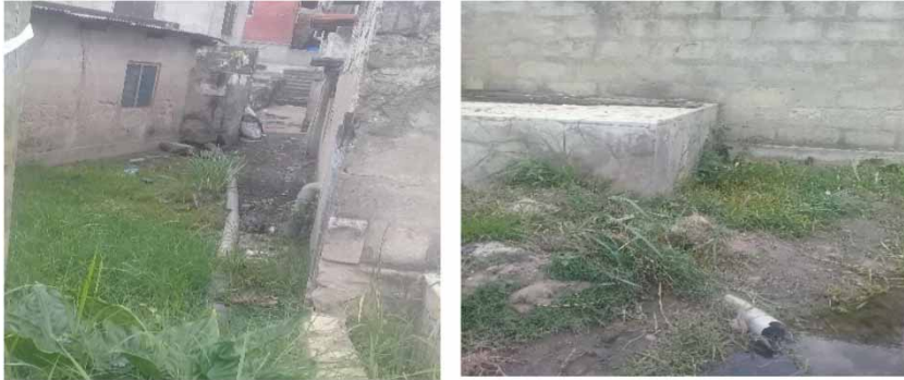
Figure 3 | Flooding out pipes connected to the toilet pits.
